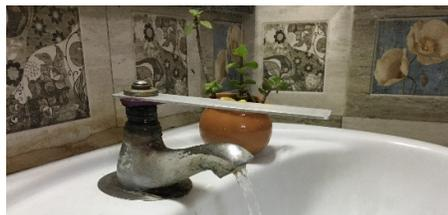
Good water flow is obtained even with 1/8 turn of regular tap. No separate installation of half-turn or quarter-turn spindles is necessitated.
